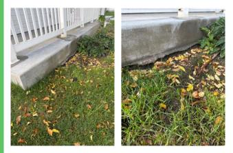
**Patios/Decks** Concrete Condition: Repair or Replace
