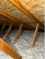
**Roof Deck Material** Oriented Strand Board Condition: Satisfactory
