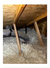
**Roof Framing Type** Wood Trusses Condition: Satisfactory
